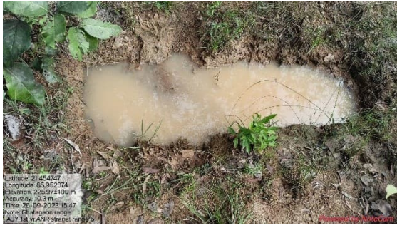
Staggered Trench, Ghatagaon, Keonjhar
