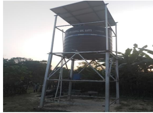
Solar overhead water Tank, Sundargarh Range of Sundargarh Division
