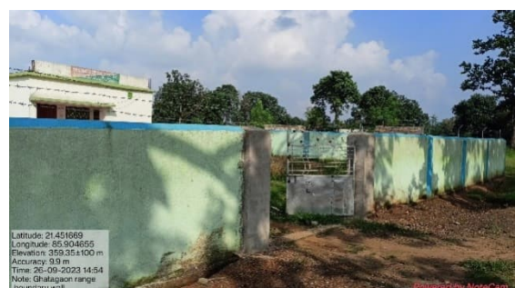
Boundary Wall, Ghatagaon, Keonjhar
